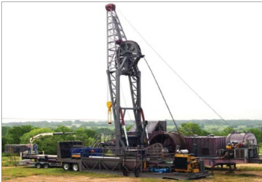
A US Department of Energy research program is using a trailer-mounted coiled tubing drilling rig with a small footprint.
