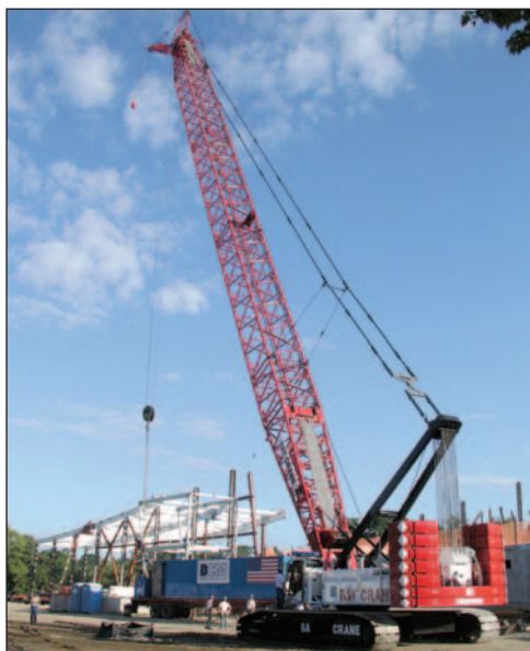
The Liebherr LR 1200 crawler crane.
