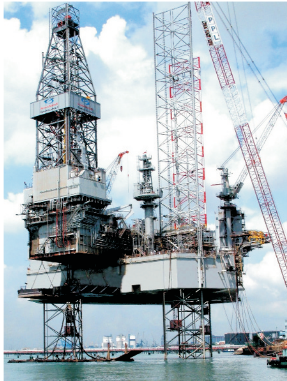
GlobalSantaFe's Constellation I as it nears completion at PPL Shipyard in Singapore. The rig is presently working for Premier Oil offshore Myanmar under a three-well plus option contract.
