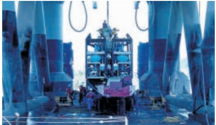
The SubSea MudLift drilling package is being lifted from the barge to the Ocean New Era in preparation for the first application of the new technology.
