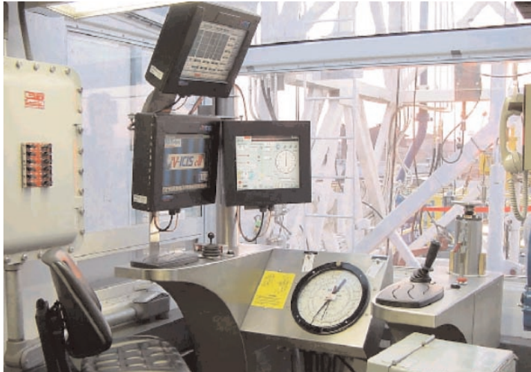
Climate-controlled driller's cabin on the latest generation FlexRig allowed addition of more electronic controls, and joystick controls for block travel and cathead operation.
