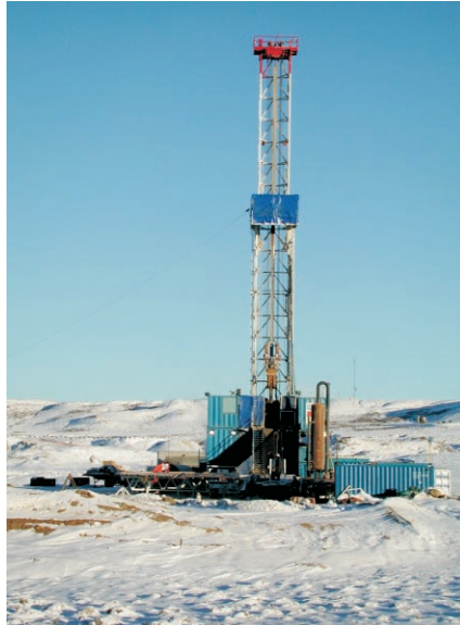
“Unconventional” drilling techniques that can cut costs include this casing drilling job.
